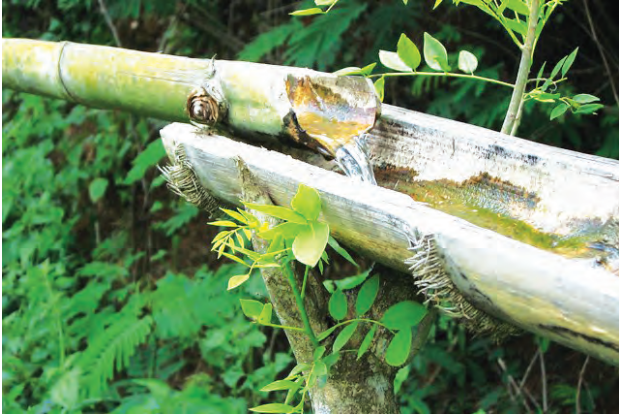
Figure 5.5 : Bamboo Irrigation System
